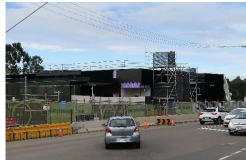
New Greensborough Station under construction, 2023. Photo B. Henderson
