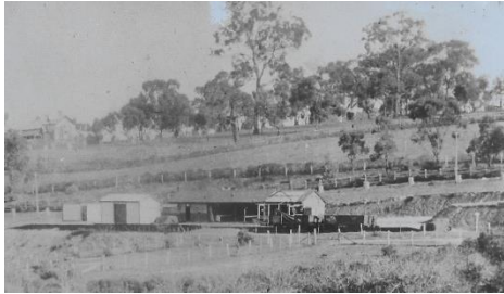
Greensborough Station, 1920s
