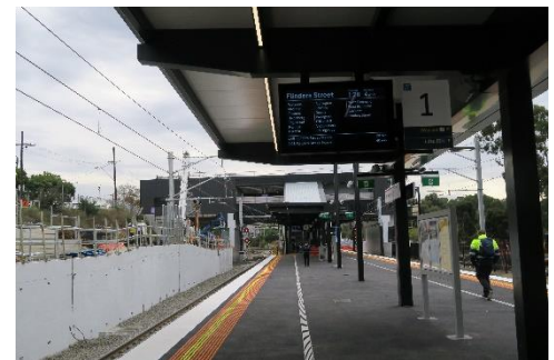
2 Greensborough Station 2023. Photo by Bryan Henderson
