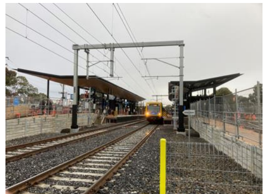
4 Montmorency Station duplicated tracks 2023. Photo by Bryan Henderson
