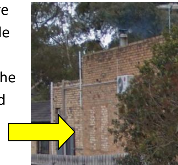
Side of shop showing bricked-in windows
